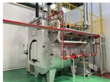
Radiant tube type hydrogen fired demonstration furnace installed at Sakai Works in April 2022
